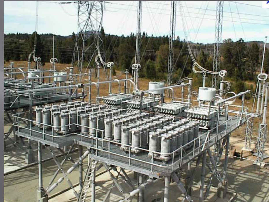
Typical series compensation (Courtesy of ABB)
