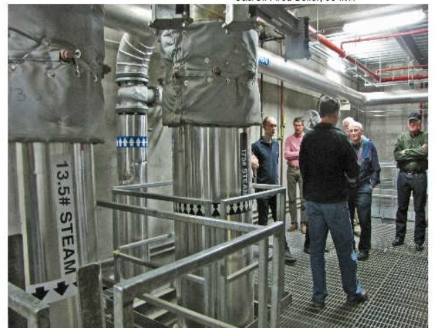
Steam Pipes to Tunnel
