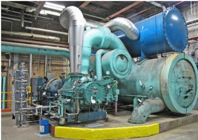
Steam Turbine Driven Chiller
