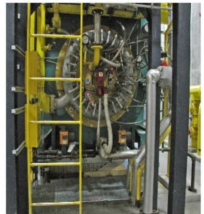
Gas/Oil Fired Boiler, 90 MW
