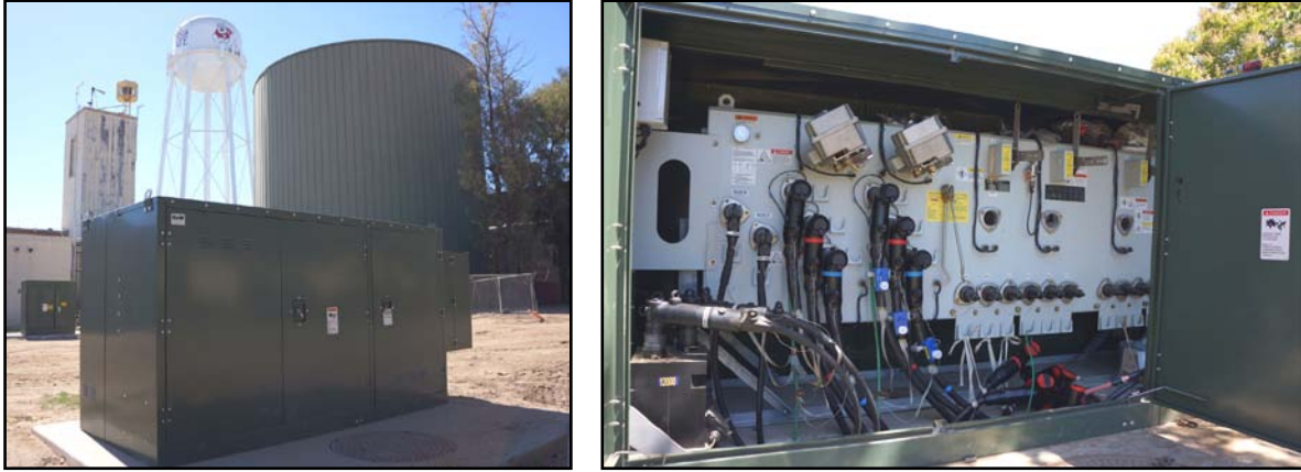
Figure 7: SF6 insulated 6-way padmount switch
