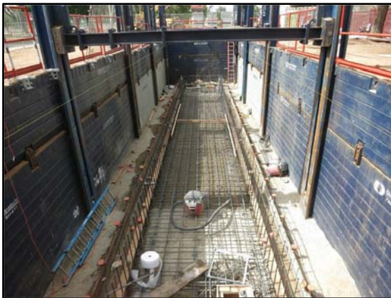
Figure 6: Cable vault below new switchgear building
