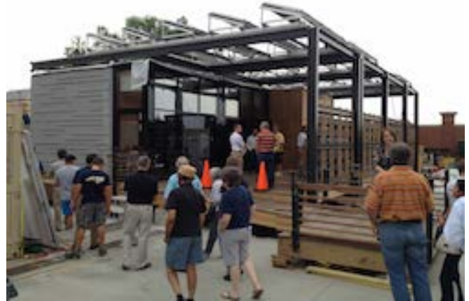
UNC Charlotte Solar Decathlon House (August 2013).
