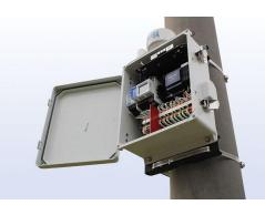
micro-PMU: Phasor Measurement Unit (PMU) for distribution applications
