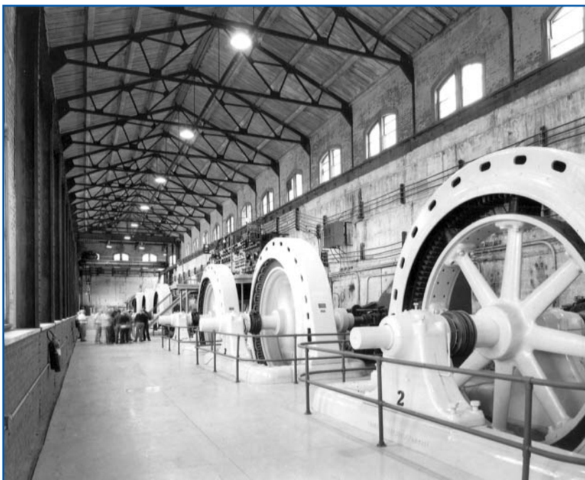
As part of the June Membership Meeting, Schenectady Section Members visited the Mechanicville Hydro Power Plant. The 4.5 megawatt plant began operating in 1898 and is on the National Register of Historic Places. – Photo Credits: Louie Powell
