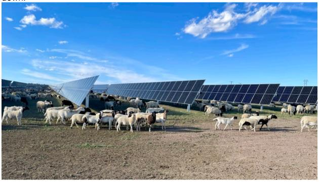
Each solar panel which is about 1 meter by 2 meters contains 144 solar cells. There are about 30 solar panels mounted on a rotating pole. The panels are series connected to create a 600 volt output.
