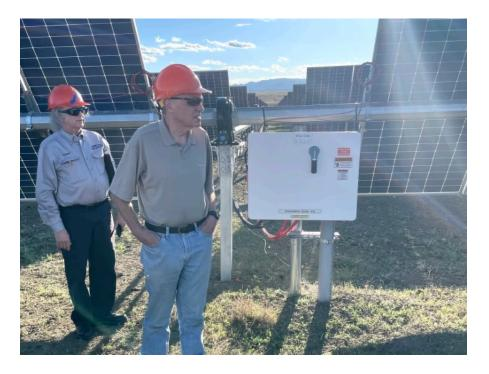
Here is the large grid-following inverter. It receives the 600 volt inputs from multiple rows of the array, convert from DC to AC voltage and up-converts this voltage to 34.5KV which is sent to a power substation nearby via buried high voltage cables. There are a total of 96 of these inverters in the overall Pike Solar Array.
