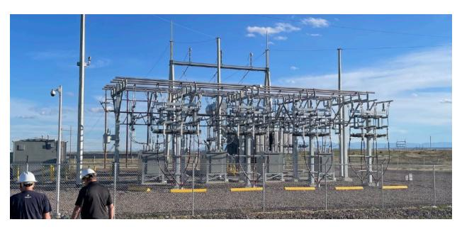
The outputs from these circuit breakers is connected to a transformer which upconverts 34.5KV to 120KV which connects the field to a nearby CSU substation which consolidates all of the solar field outputs and send the power to Colorado Springs via two major transmission lines.
