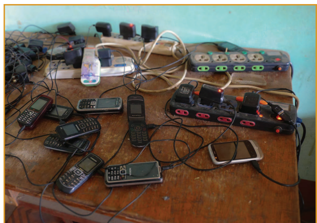
figure 4. Mobile phone recharging provides an income stream—usually US$0.25 to US$0.50 per recharge—that can help make off-grid systems economically sustainable (photo courtesy of Peter Dauenhauer).
