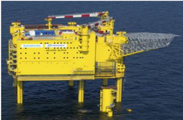
Offshore Converter Station
