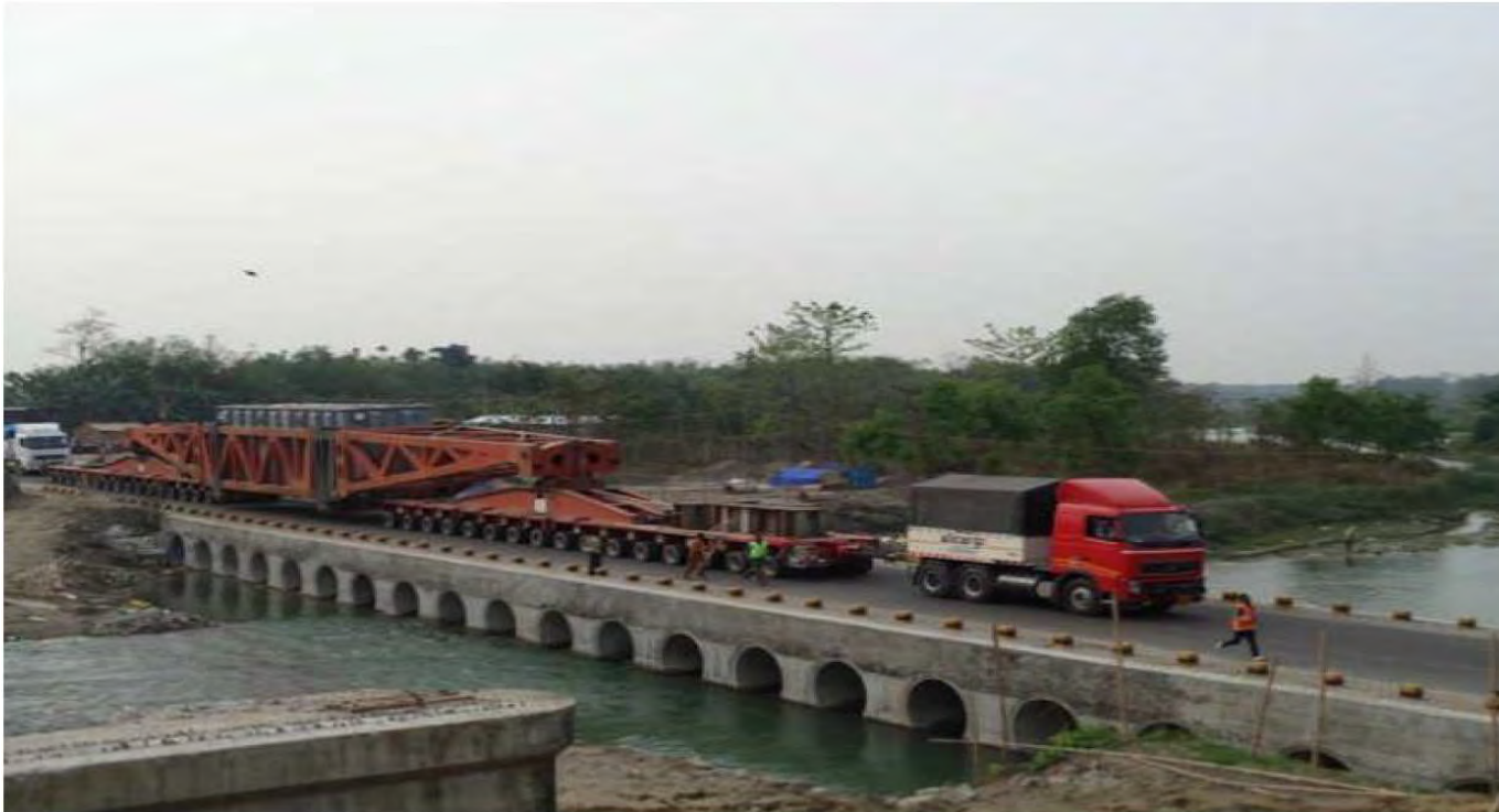
Transport to APD of 800 kV transformer on girder bridge over a by pass (temporary bridge)
