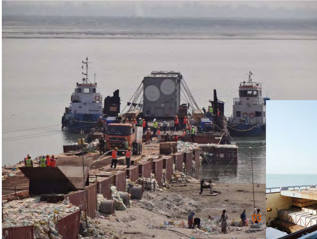
▪Transformer under unloading at the jetty
