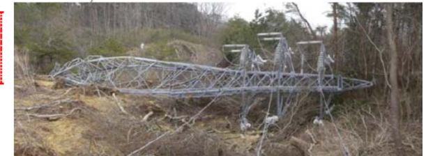
Collapsed pylon
