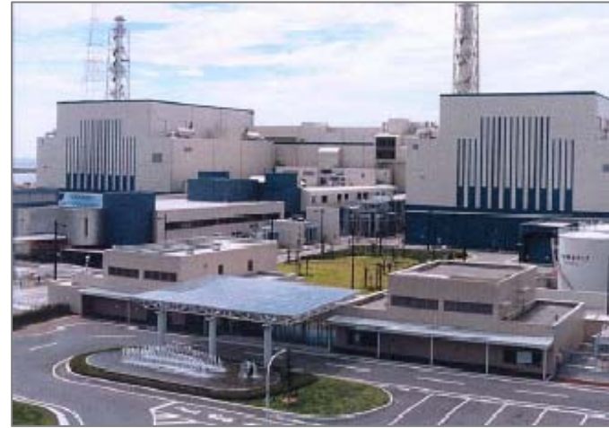
ABWRs Being Built in Japan
