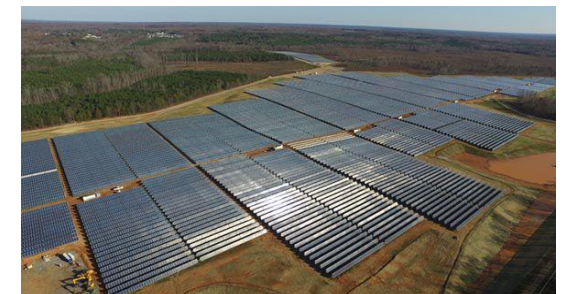
Dominion Energy Scott Solar Facility (Source: Richmond Times Dispatch)
