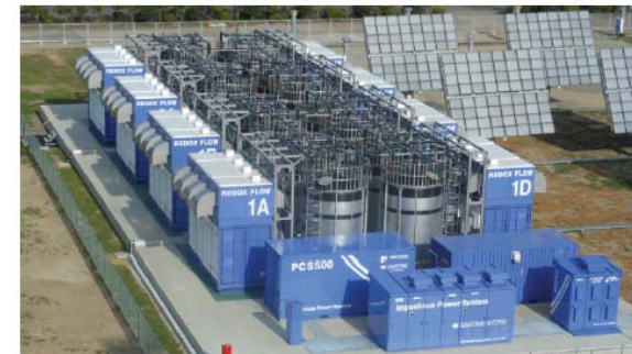
Aerial view of the 5-MWh RFB and 100-kW PV.
