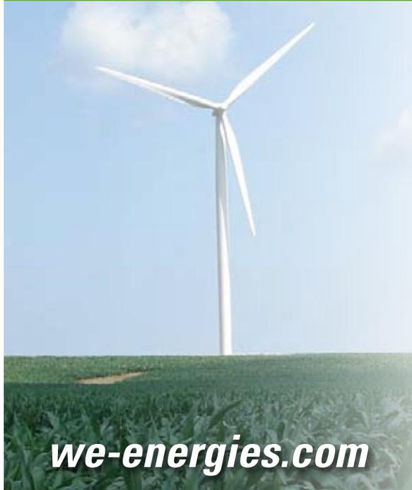
The Blue Sky Green Field Wind Energy Center, located in the towns of Calumet and Marshfield in northeast Fond du Lac County, is designed to generate 145 megawatts (MW) of electricity, and is capable of powering approximately 36,000 average residential homes. The site consists of 88 wind turbines.
