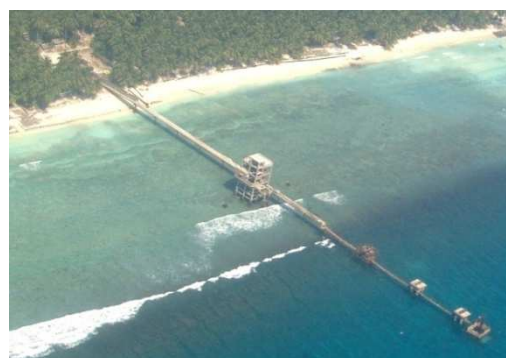
Fig.6. Desalination plant in Agatti Island of India
