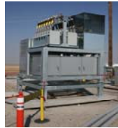
Emprimus Transformer Neutral Blocking System
