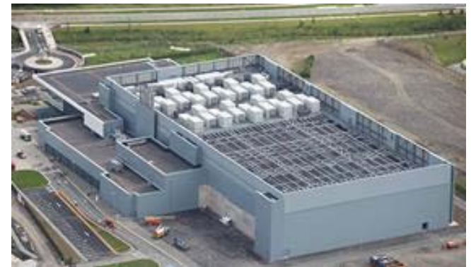
Microsoft mega scale data center, Dublin, Ireland (opened 2009)
